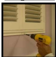
Only secure one screw into the bottom frame.
