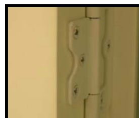
Hinge spacer installed
