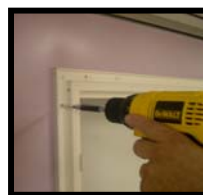
Only secure one screw into the top left frame.
