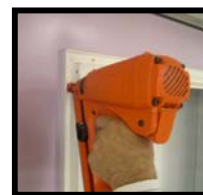
Only secure one nail into the top left frame.
