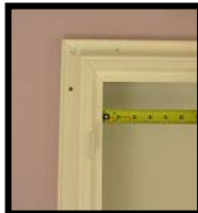
A tape measure can help space your shutter evenly around window.
