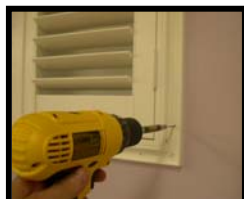
Only secure one screw into the bottom right frame.
