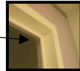
Only secure one nail into the top left frame.
