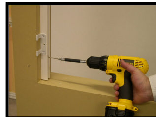
With hinge lined up, secure the bottom screw into the pre-drilled hole.
