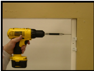
With hinge aligned, secure the top screw.
