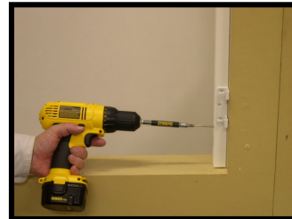
With hinge lined up, secure the bottom screw into the pre-drilled hole.
