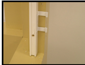
Once top screw is tightened, line up the bottom hinge in reference to top hinge position.
